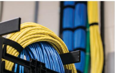
Belden 10GXS Category 6A cable was used to establish two drops in each classroom across the Forsyth County Schools district. By pulling two cables, the district now has redundancy. If one switch fails, a second switch keeps things running.
